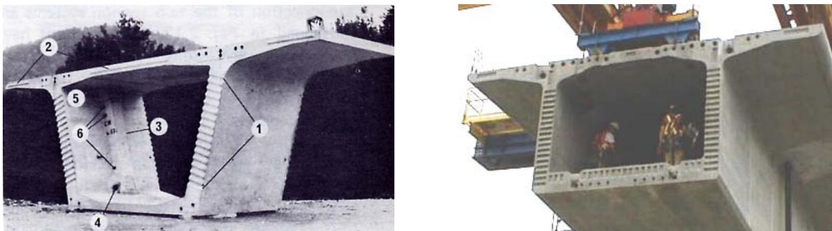
**Figure 1** Precast segmental box girder sections. Left: pre-1975 (PTI 1978). Right: 2000
