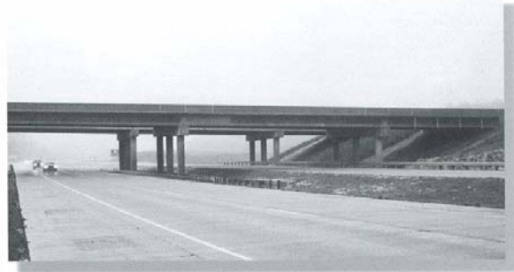
The use of high strength concrete allowed wider girder spacing.
