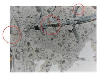
*Fig.* 12—*Corrosion spotted on reinforcing bars.*
