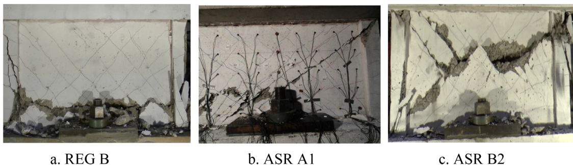
Fig. 5. Regular and ASR walls at failure.
