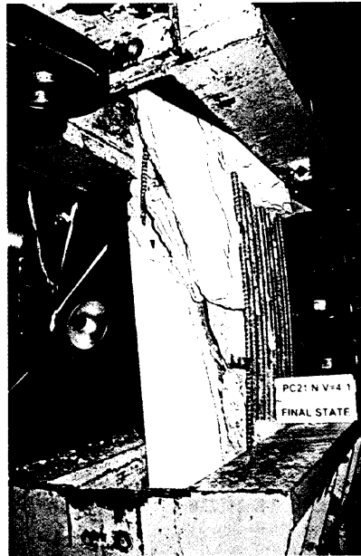
Fig. 16 — Reinforced concrete wall after failure.
