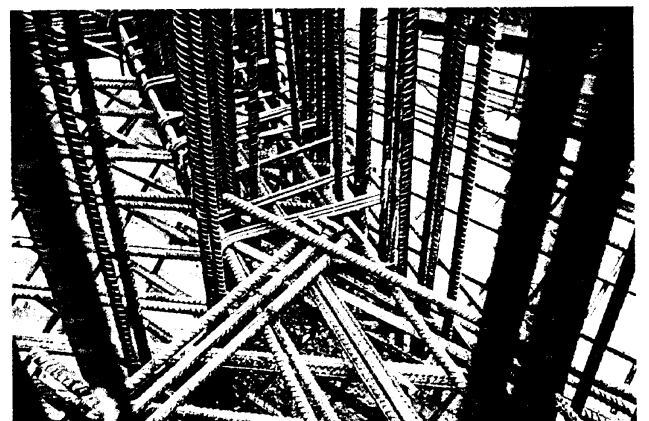
Fig. 8 — Placement of T-headed bars across the throat of the tricell.
