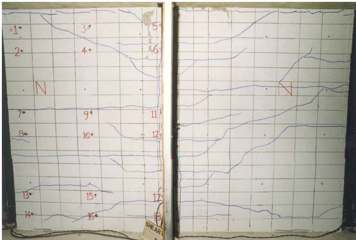
Figure 5-19 Crack pattern and damage sustained by the flange of Palermo shear wall DP2 at the termination of the test (Palermo, 2002)
